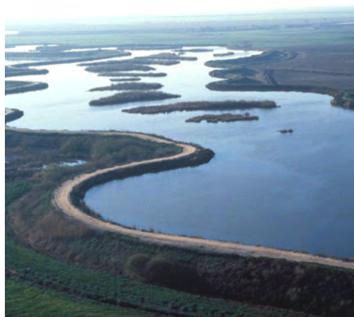
Photo courtesy of The Metropolitan Water District of Southern California.
