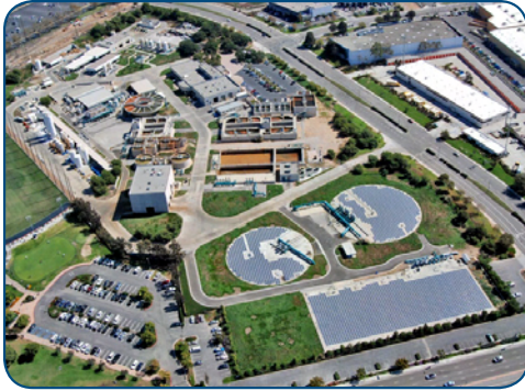
Edward C. Little Water Recycling Facility
